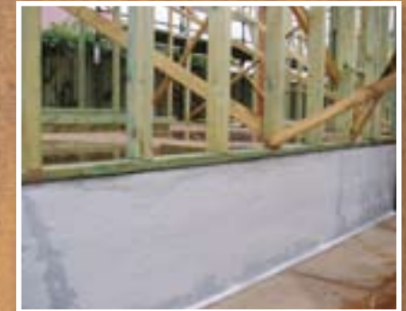
Delta Blanket Retaining Wall
