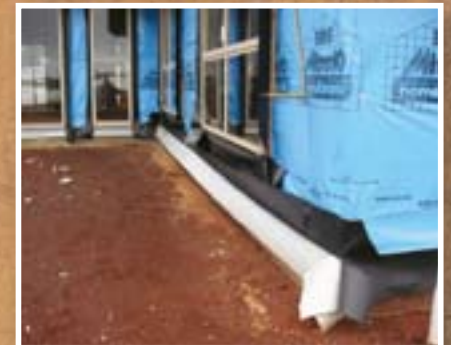
Perimeter (under frame)
